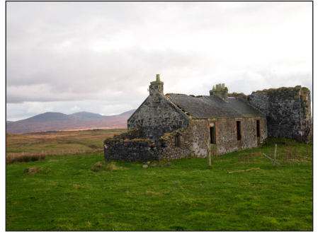
Fig. W7.27 The engine house at Mulreesh.
